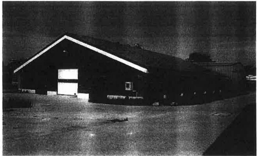
Figure 1 Natural ventilated experimental cattle livestock building with eaves to ridge ventilation
