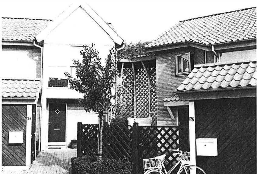
Figure 8. Two-storey wind shield and the southern facade of a house with the living room on the first floor
