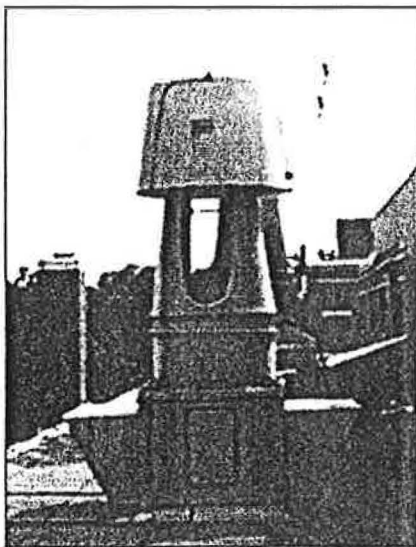
5 The bi-furcated fan design allows fresh air to be aspirated into the contaminated air stream as well as through the stack shroud, thereby encapsulating the contaminated air in the exhaust plume and allowing the stack to be shortened.
