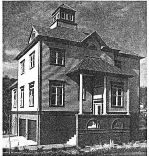
The HVAC equipment in the 3200 ft 2 , four-story house is located on the second floor, reducing the amount of ductwork needed.
