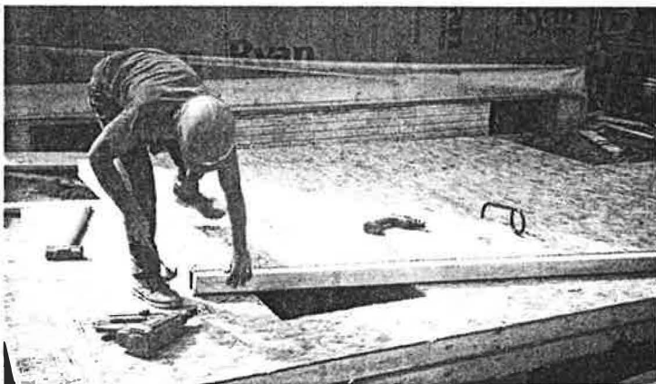
Structured insulated panels (SIPs) were used in CARB's Building America homes whenever appropriate because of the speed and ease of construction, because they contain renewable resources, and because of their high R-values.
