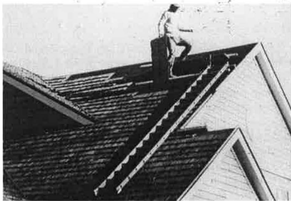
Figure 3 Plastic shake roofing (w/skylights).
