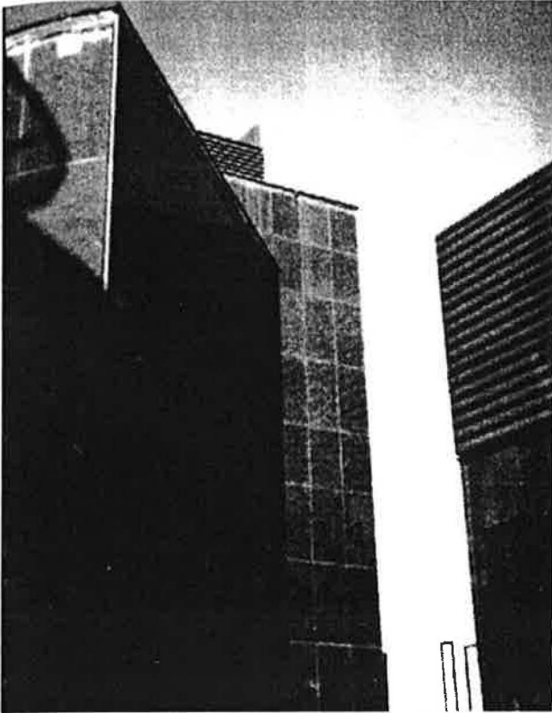
Figure 5 – External view of two vents.
