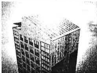
Figure 5: View of new roof.
