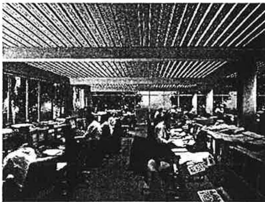
Figure 6: Composite deck - exposed soffit
