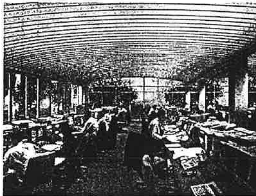
Figure 8: Exposed soffit with curved metal decking (N.B. last structural bay may require ties)
