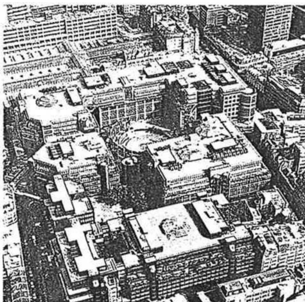
Fig. 6.1.1 Total view of the Broadgate City Complex
