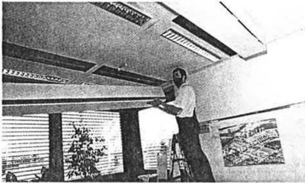
Fig. 6.12.3 Installation of the “cooling girders“
