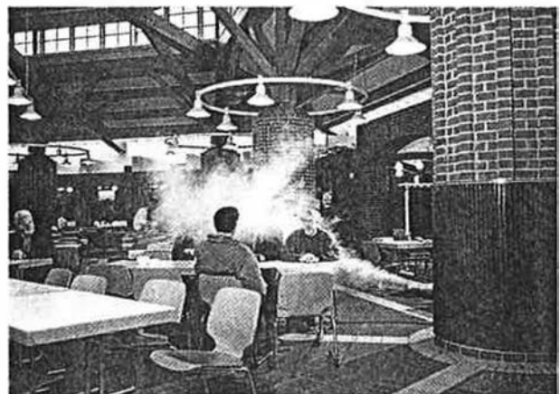
Fig. 2.2.2.1 Air terminal device for source ventilation in a casino (5)
