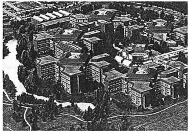
Fig. 6.2.1 Total view of the building complex
