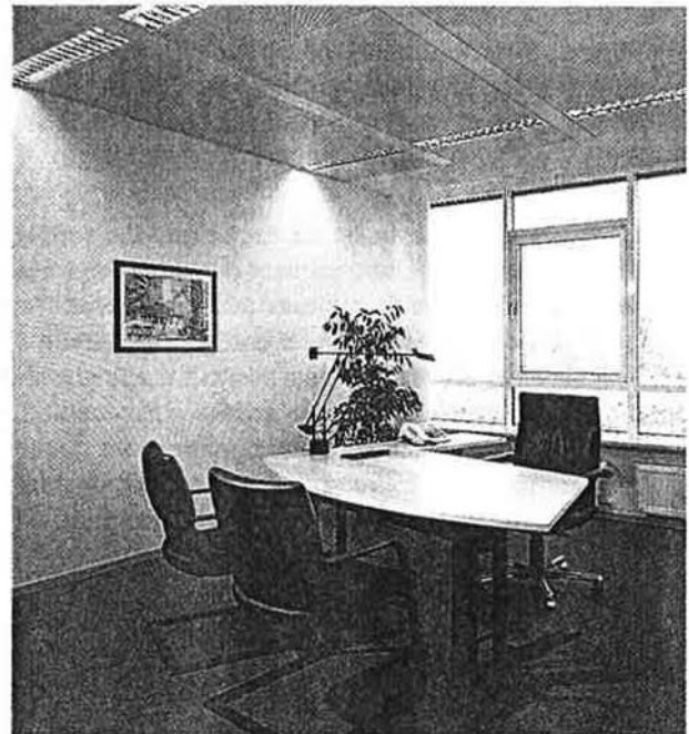
Fig. 6.7.3 View of the ceiling in an office
