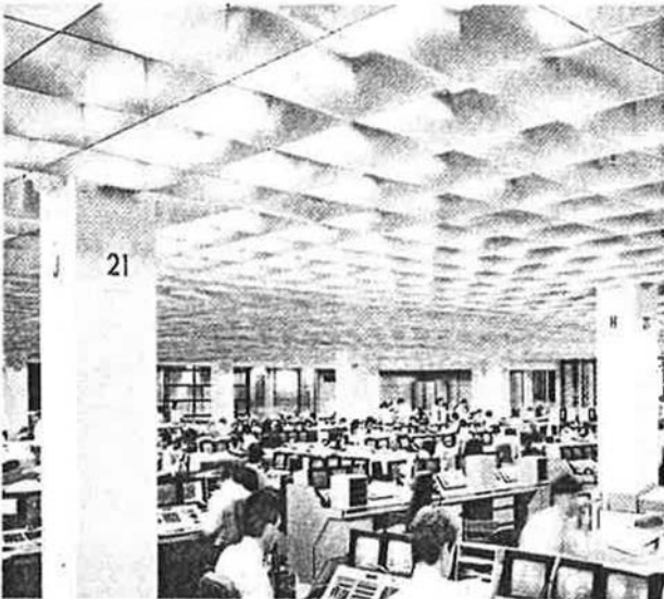
Fig. 6.1.3 Work area of the foreign exchange and security dealers with mirror section grid ceiling
