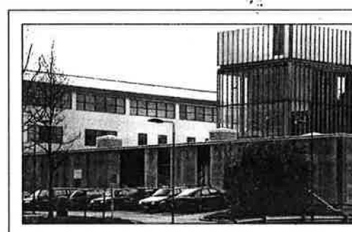
Hertfordshire University has installed Monodraught's Windcatcher natural ventilation in two lecture halls in an attempt to reduce energy costs.
