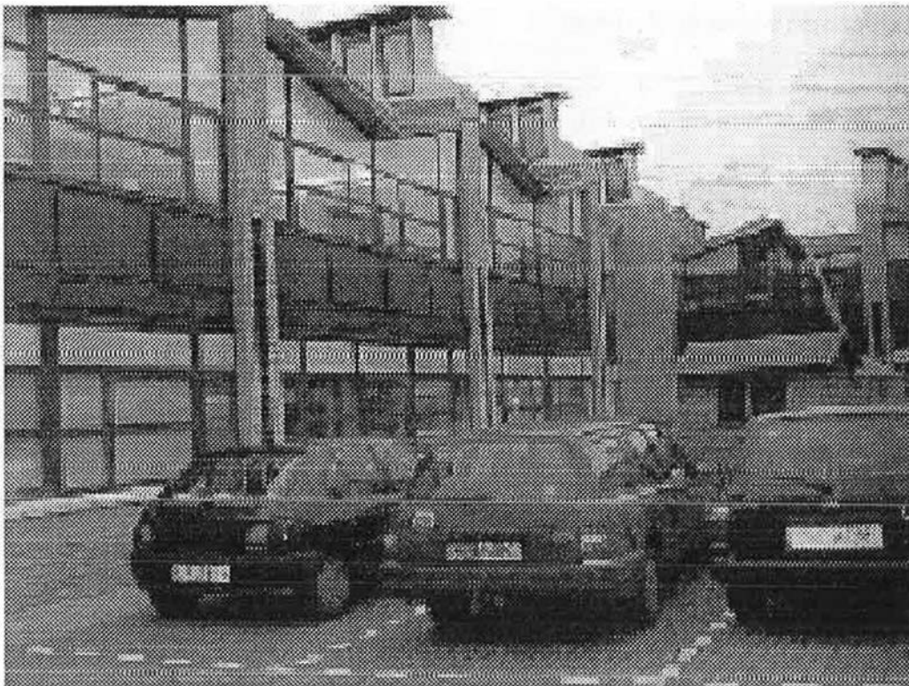
Figure 1(b). View of the Canning Crescent Centre from the Courtyard Side.
