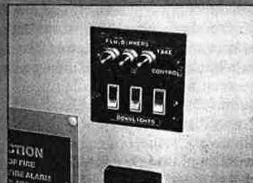
Note the clear and concise labelling of the building controls.
