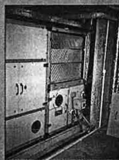
The heat recovery systems for two of EFry's air handling units use high-efficiency heat exchangers. These are claimed to recover 85% of the available heat, a figure verified by the monitoring.
