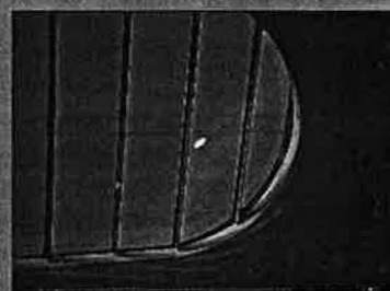
The rooflights above the stairs show a slight tendency towards air leakage.
