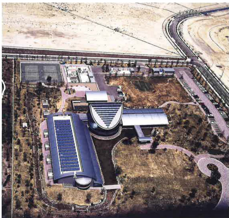
Photo: Aerial view of RITE's Home Laboratory.
