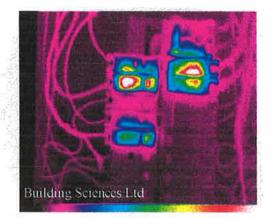
Again thermography can be employed to quickly assess the performance of individual circuits by scanning the fuse boards. Overloaded fuses are seen here with white centres. The overloaded circuit heats up and can threaten fires if connections are poor.
