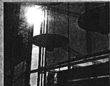
Sun glare into the reception area required a retrofitted sunblind.
