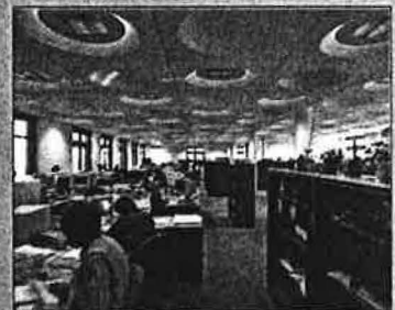
The project architect for the CAF building provided a high quality exposed ceiling-scape into which the services engineer integrated the lighting, but...
