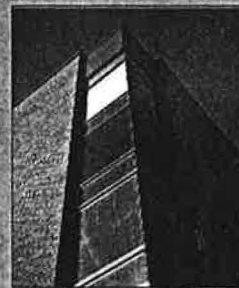
ABOVE: Despite the lack of a pressure test, evidence of uncontrolled infiltration was easy to find using a smoke pencil, specifically around the edges of the planar windows, LEFT.
