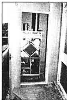
ABOVE, FIGURE 2: The Genvex units consist of a large heat pump unit and two fans – supply and extract – at the top. For the two-bedroom flats, the Genvex mvhr units were located on enclosed balconies, LEFT. This reduced the length of the inlet and extract ductwork, and simplified the disposal of condensate waste.
