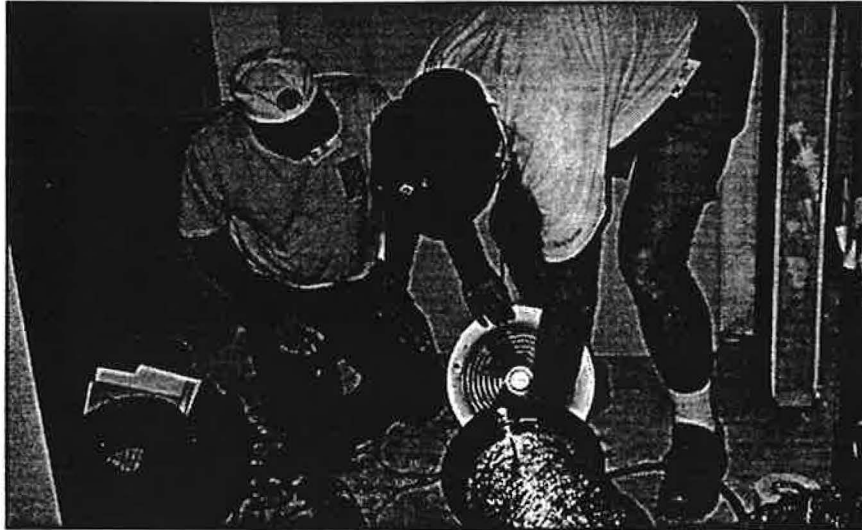
Figure 6. Energy specialists demonstrated methods of measuring energy efficiency to volunteers during the week of construction. Here, a duct test revealed a large duct leak that was sealed in this and subsequent houses.
