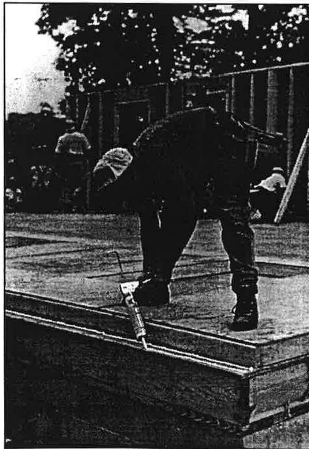
Figure 5. Energy specialists at each construction site made sure energy-efficient construction practices were followed, especially at the beginning of construction when caulking was required before walls were raised.
