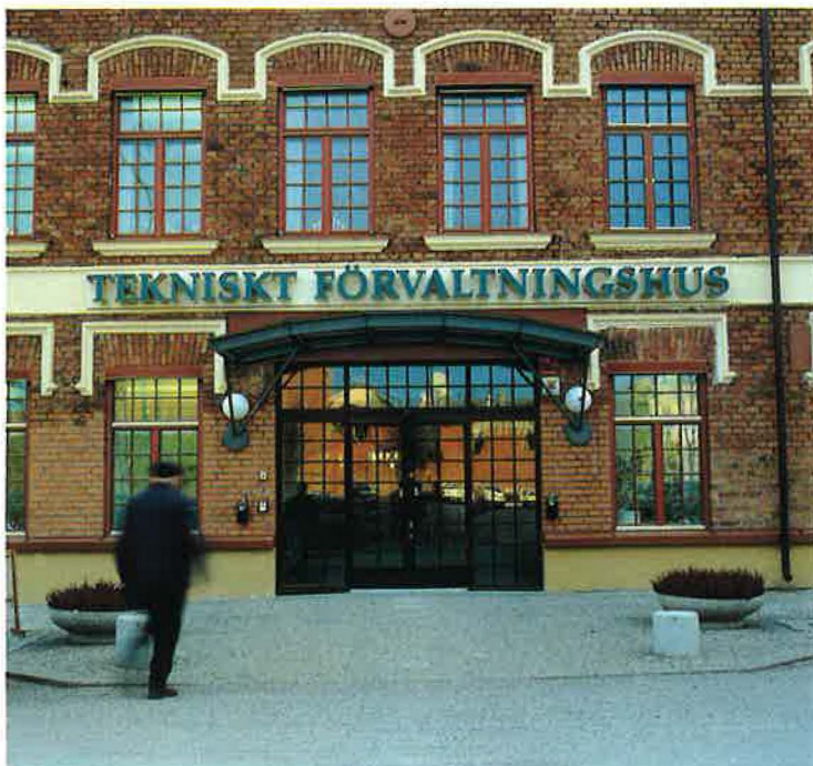
The retrofitted building in Eskilstuna.
