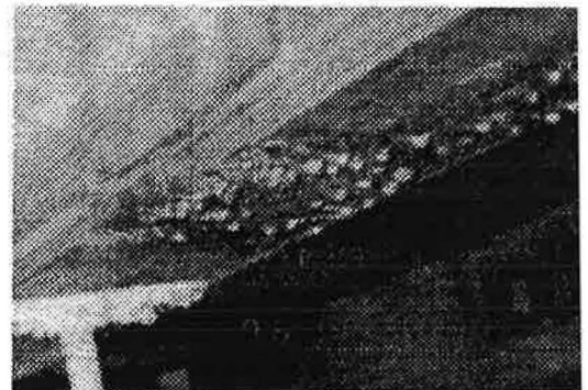
Figure 4 Water drops on surface of floor joist
