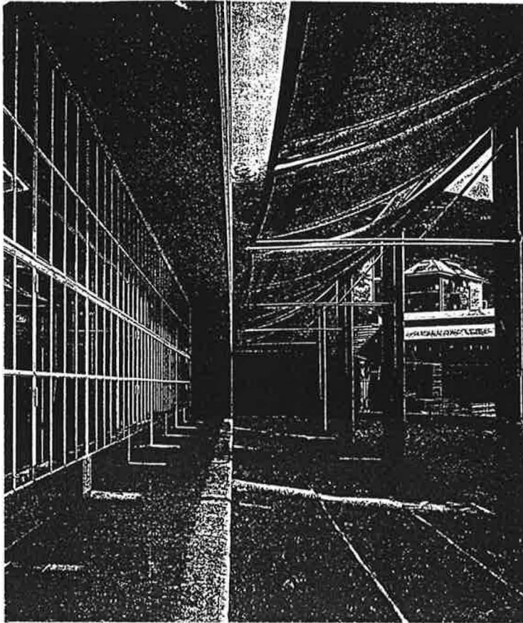
FIG. 15 Combination of fixed and movable shading at Asilo Sant'Elia (G.Terragni).
