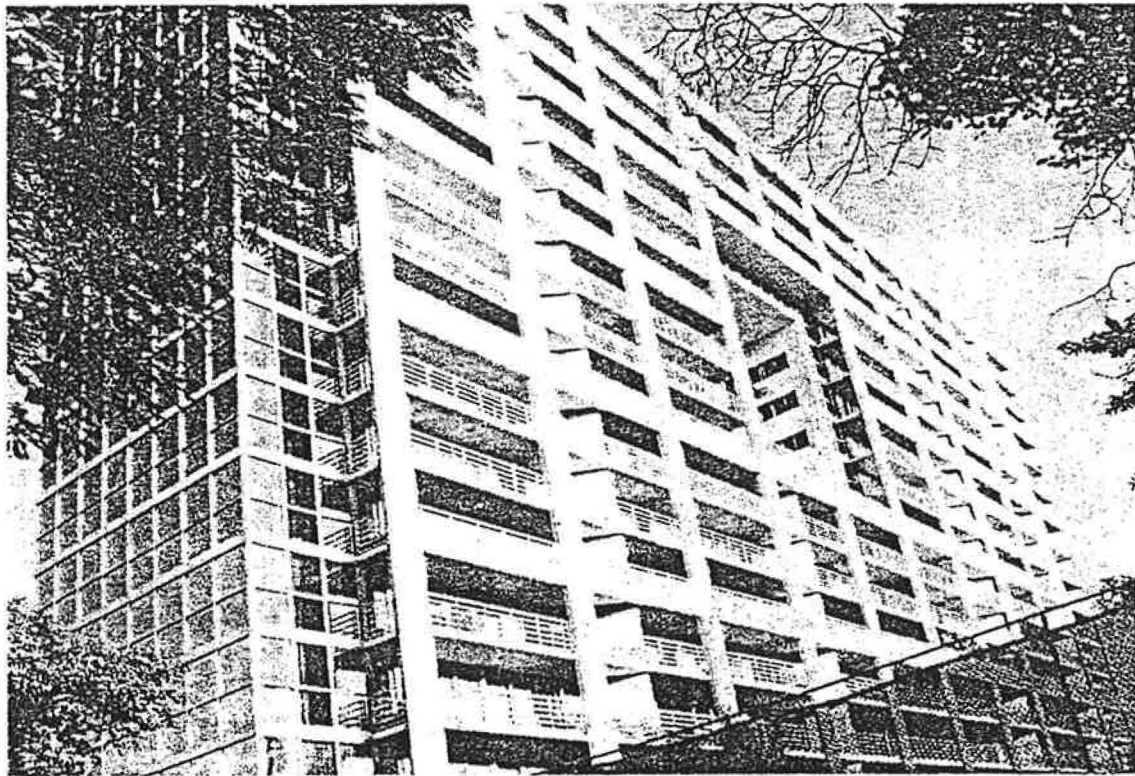
FIG. 3 Combination of solar control modes
