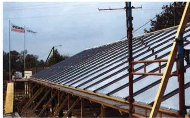
ONSA LA IN GÖTEBORG (SWEDEN) – PREFABRICATED ROOF MODULE WITH INTEGRATED SOLAR COLLECTORS
