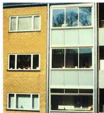
KILDEPARKEN, COPENHAGEN (DENMARK) – GLAZED BALCONIES AND TRANSPARENT INSULATION IN PARAPETS
