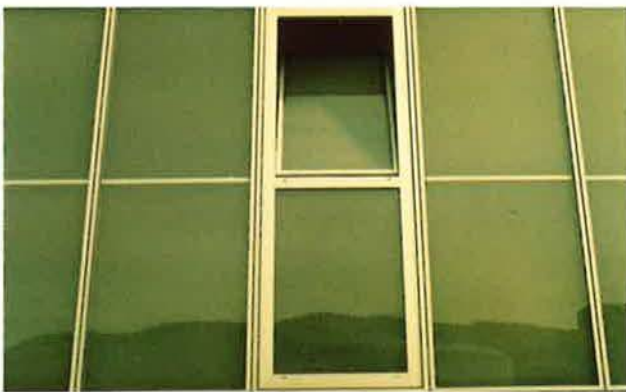
LABORATORY PSI (SWITZERLAND) – TI AS DAYLIGHTING ELEMENT
