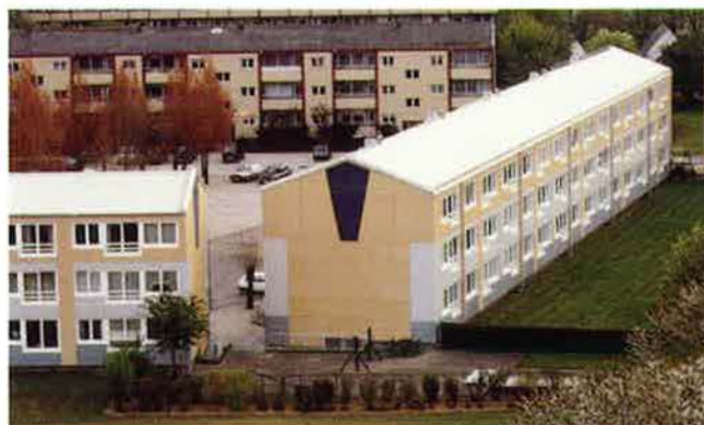
HYBRID SOLAR HOUSE, COPENHAGEN (DENMARK) – ROOF COLLECTORS FOR HEATING THE CAVITY WALL
