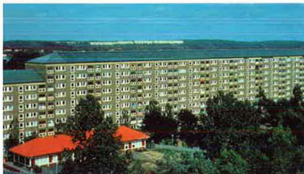
HAMMARKULLEN IN GÖTEBORG (SWEDEN) – ROOF COLLECTORS FOR DHW
