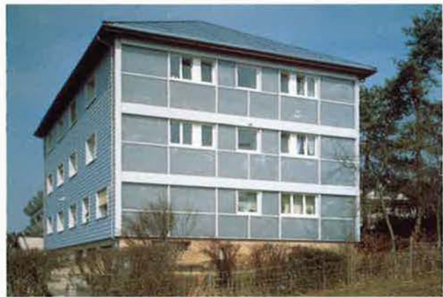
AFFOLTERNSTRASSE, HEDINGEN (SWITZERLAND) – BEFORE RENOVATION AND WITH SOLAR RENOVATION: A TI WALL IS USED FOR HEATING AND ROOF-INTEGRATED SOLAR COLLECTORS FOR DHW
