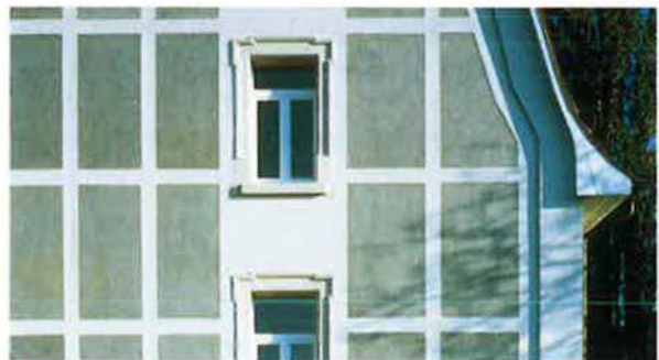
VILLA TANNHEIM IN FREIBURG (GERMANY) – COMPOSITE TI/PLASTER SYSTEM
