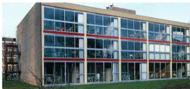
ELVIRA IN AMSTENRADE (THE NETHERLANDS) – GLAZED BALCONIES IN SENIOR CITIZENS' APARTMENTS
