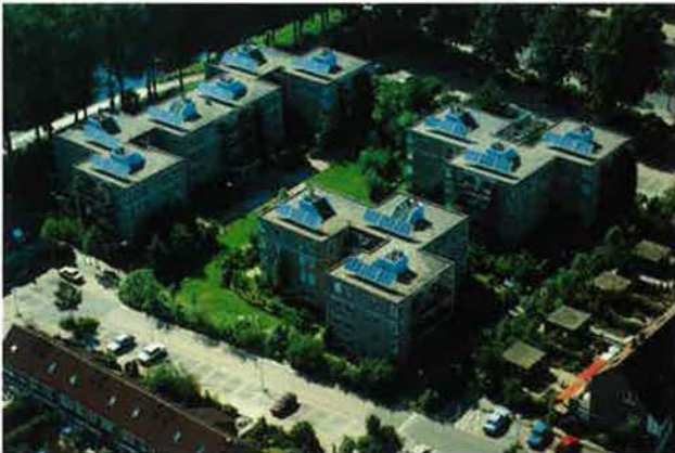
KLOPVAART, UTRECHT (THE NETHERLANDS) – SOLAR COLLECTORS FOR DHW
