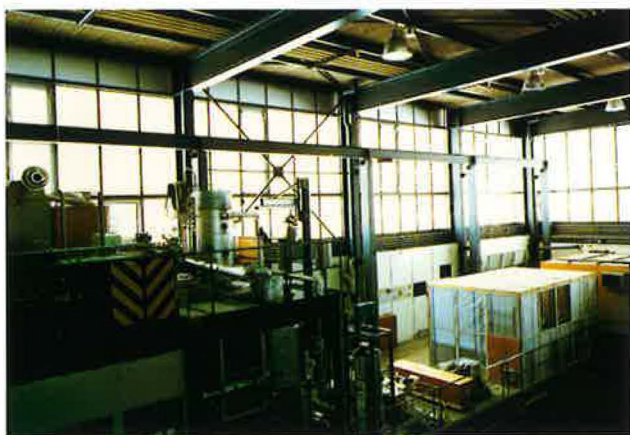
THE OVERALL RENOVATION OF A LABORATORY BUILDING INCLUDED REPLACEMENT OF THE SINGLE-GLAZED FACADE WITH TI GLAZING ELEMENTS. (LABORATORY BUILDING AT PAUL SCHERRER INSTITUTE, WÜRENLINGEN, SWITZERLAND; PROJECT: M. ERNI)
