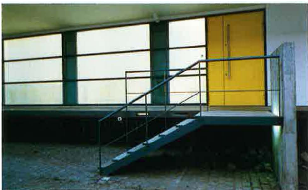
IN A CONVERSION OF AN OLD WAREHOUSE TO AN OFFICE BUILDING OPAQUE WALLS HAVE BEEN REPLACED WITH TI GLAZING TO ILLUMINATE MEETING ROOMS. (WWF HEADQUARTERS SWITZERLAND, ZÜRICH; PROJECT: COLE+ZIMMERMANN)
