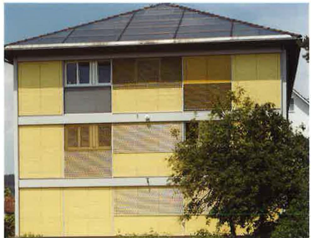
TI FACADE SHADED WITH EXTERNAL VENETIAN BLINDS
