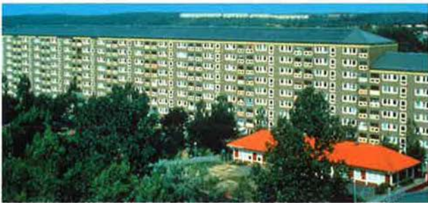
ROOF-INTEGRATED SOLAR COLLECTORS
