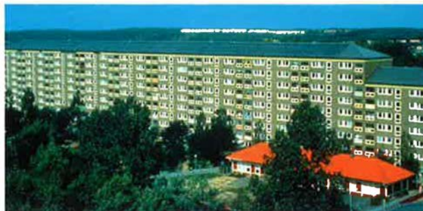
ROOF-INTEGRATED SOLAR COLLECTORS
