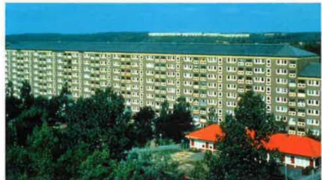
ROOF-INTEGRATED (SITE-BUILT) COLLECTORS ON A MULTIFAMILY BUILDING IN GÖTEBORG (HAMMARKULLEN), SWEDEN
