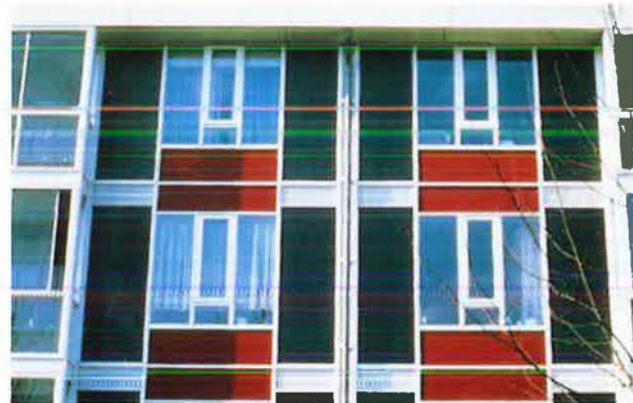
FACADE-INTEGRATED SOLAR COLLECTORS AND GLAZED BALCONIES
