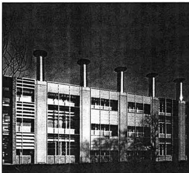
Integrated environmental design in action. The South facade of this project at the Building Research Establishment clearly shows the ventilation stacks and motorised solar-control louvres. This photograph shows how the louvres can be positioned to provide protection from sunlight or to admit light to maximise the use of daylight.
