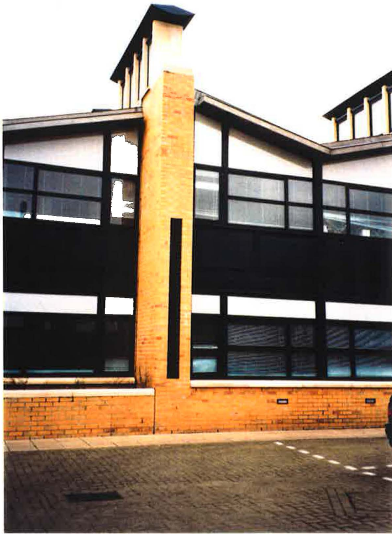
Stack Intake grill from courtyard
