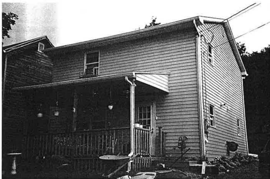
Pictured here is the most efficient home built by Greene County Pennsylvania's Habitat for Humanity affiliate. The purchase price was $30,000, which included the in-kind value of the property and donated materials, as well as a $3,000 administration fee. The family contributed well over the 500 hours of sweat equity required of Habitat homeowners.
