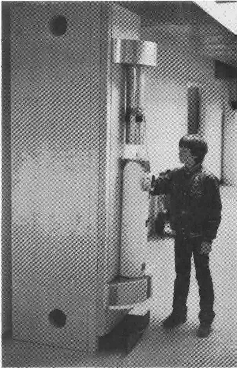
FIG. 11 Air-to-Air Heat Exchanger built from plans developed by Besant [7] at the University of Saskatchewan.
