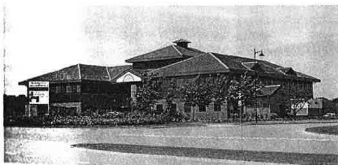
Figure 1 The United Kingdom's first FES-slab building (Weidmüller Klippon Microsystems at West Malling, Kent)
