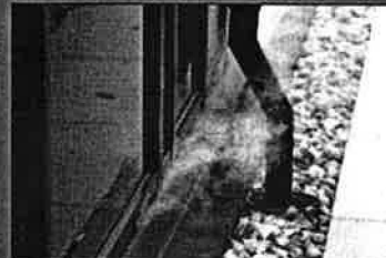
Gardner House: air leakage seriously affected fuel efficiency and comfort levels.
