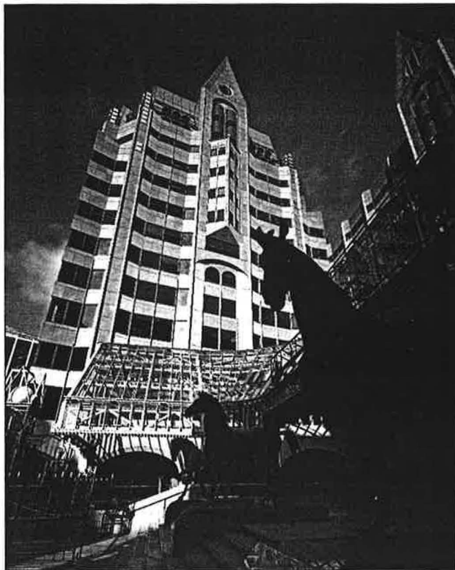
Minster Court, owned by Prudential Portfolio Managers, is a group of three large multi-tenanted buildings with mechanical services designed by Ove Arup & Partners. The plant consists of multiple vav terminals on each floor supplied by local packaged ahus.
