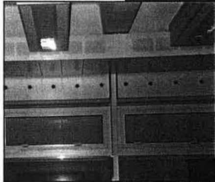
RIGHT: A typical office floor prior to tenant fit-out. Note the Trox service beams installed between the ribbed coffers, the openable windows and the perimeter heating. INSET: Close-up of the permanent circular trickle vents, sized at 160 cm 2 per 3 m bay. Overall, the architectural integration could have looked better.
