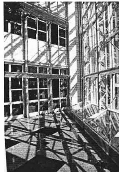
Inner view of one atrium with the air outlets in the floor. In the back are the office windows with the solar protection discernible.
