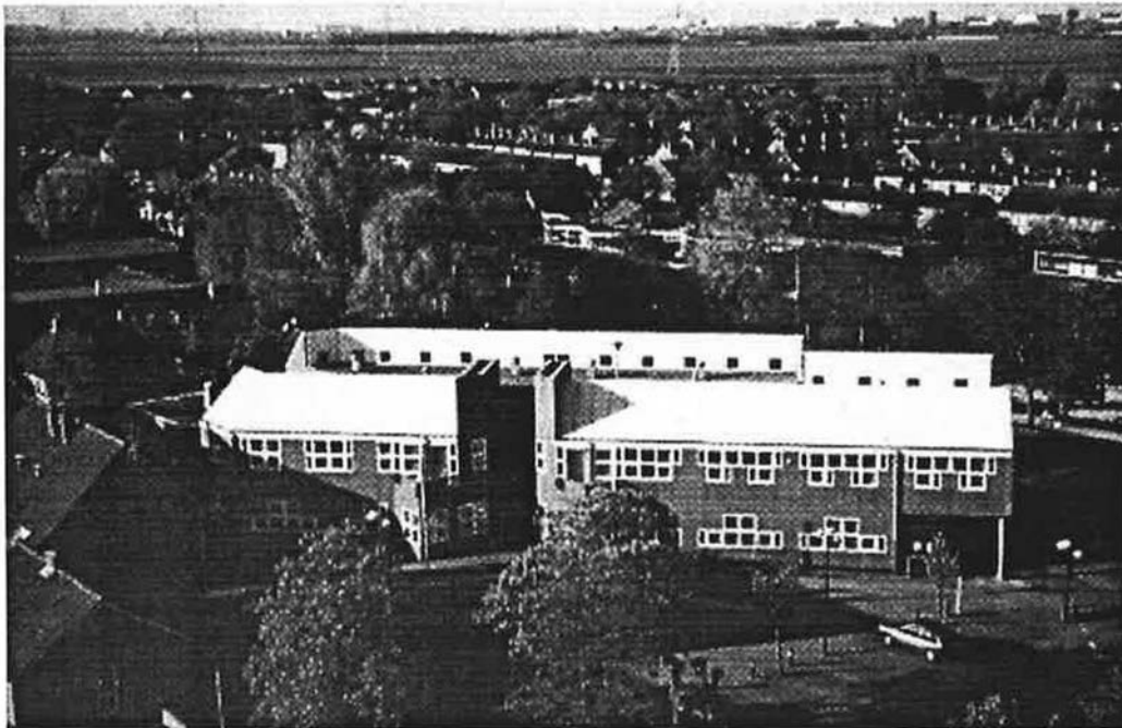
The Townhall of Zevenhuizen-Moerkapelle
