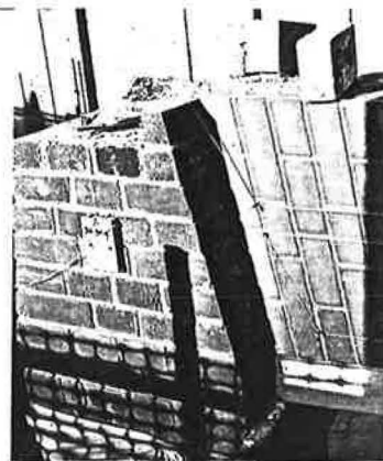
4. Brickwork detail on arch.
