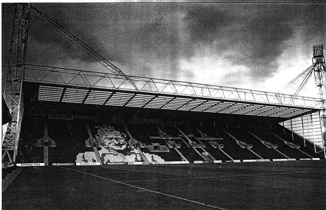
▲ The new stand at Preston North End Football Club bears that name of its most famous player, Tom Finney. As well as being a soccer legend, Mr Finney also founded a building services contracting company which was the one chosen, appropriately, to carry out the m&e services including Andrews water heaters and Chaffoteaux boilers to supply hygienic hot water.
