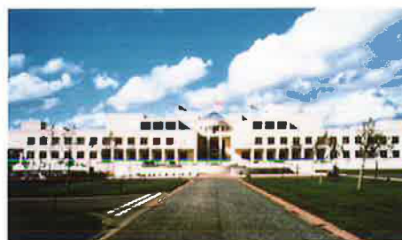
NFU Mutual and Avon Group Head Office designed to avoid air conditioning in most areas
