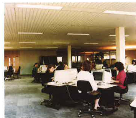
This office with high frequency lighting has an installed load of 8.5 W/m 2 (as against typically 15-20 W/m 2 ) and includes automatic dimming for further savings.
