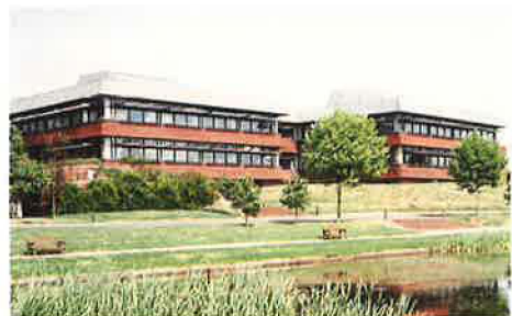
At Hereford & Worcester County Hall new lamps and reflectors now allow one fluorescent tube to do the work of two old ones, using less than half the electricity.
