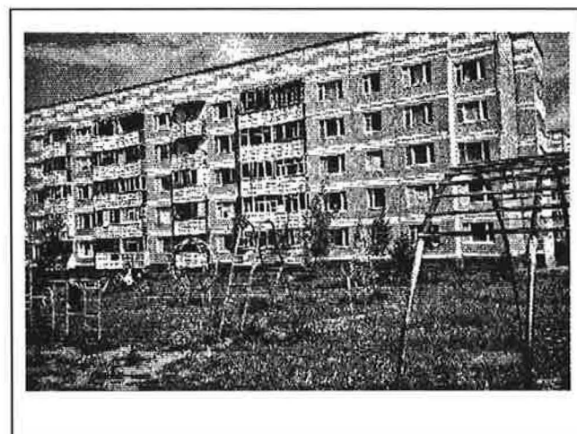
Figure 5. 5-Story Demonstration Building
