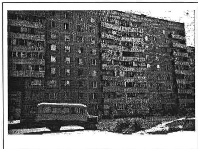
Figure 4. 9-Story Demonstration Building
