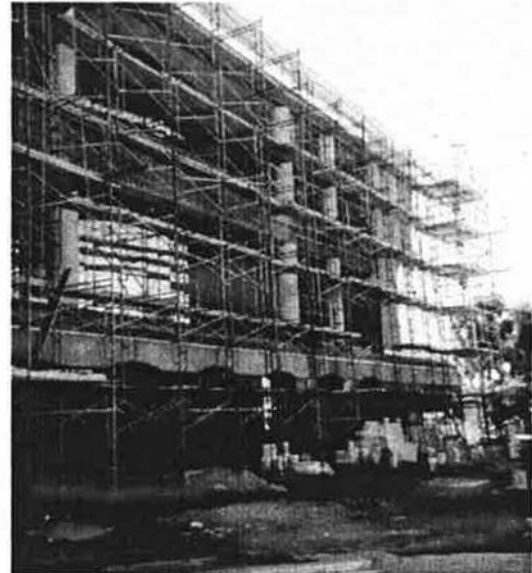
Figure 1-1. Although brand new, this municipal building was evacuated shortly after it opened because occupants were reporting health complaints. Mold and mildew were the culprits, and in the end, the problem will require more than $20 million to repair.
