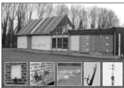
Measurement set-up for wind, rain and wind-driven rain. Main figure: South-west facade of the VLIET test building equipped with 20 wind-driven-rain gauges (white squares). Details (from left to right): wind-driven-rain gauge on building facade, rain-water reservoir at inside of building facade, rain-gauge installation, meteorological mast situated 20 m south-west of the building, ultrasonic anemometer on top of mast.
