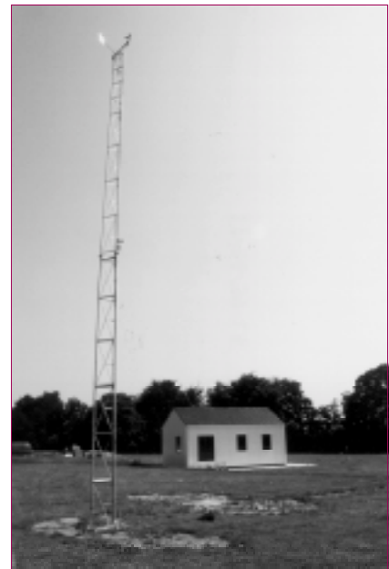
Test house on the site of BBRI (Limelette - Belgium)
