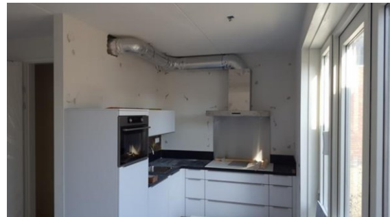
Figure 5: Range hood with reduced pressure drop and 180 mm diameter noise reducing duct
