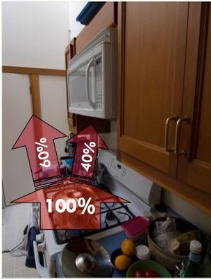
Figure 3: Capture efficiency of a range hood commonly found in the U.S.A (Image courtesy of Iain Walker at the Lawrence Berkeley National Laboratory).
