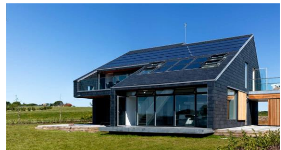
Figure 3: Solstad, Larvik, Norway. Kindergarten in Norway with hybrid ventilation combining motor controlled operable windows with balanced mechanical ventilation.
