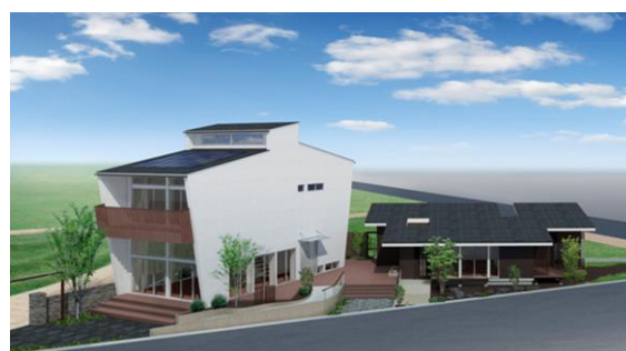
Figure 8: M-smart city Kumagaya, Kumagaya-shi, Japan. Exhibition House, Japan. Openings' orientation to prevailing wind, shape of balconies and monitored roof openings facilitate cross and stack ventilation.
