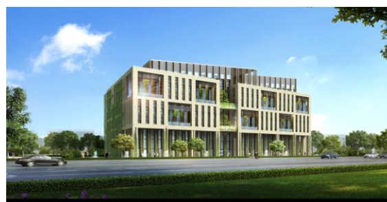
Figure 7: Franshion Exhibition Centre, Changsha, Hunan Province, China. The building uses concave balconies defined by an electric sunshade glass louvre so that the building shape coefficient can be changed in different.
