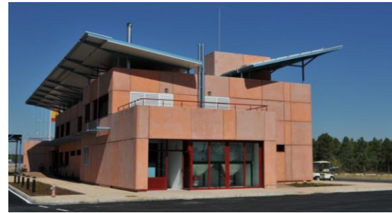
Figure 2: C-Ddl ARFRISOL CEDER, Altos de Lobia, Soria, Spain. Retrofit of office building using cross ventilation and intake chimneys, evaporative pads on top of windows, ventilated pergola on roof with solar thermal collectors and direct evaporative systems inside the Air Handling.
