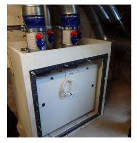
Figure 3-6 Central unit with fire protected housing and fire dampers at the top. The fire protected maintenance cover at the front is not mounted at the moment.
