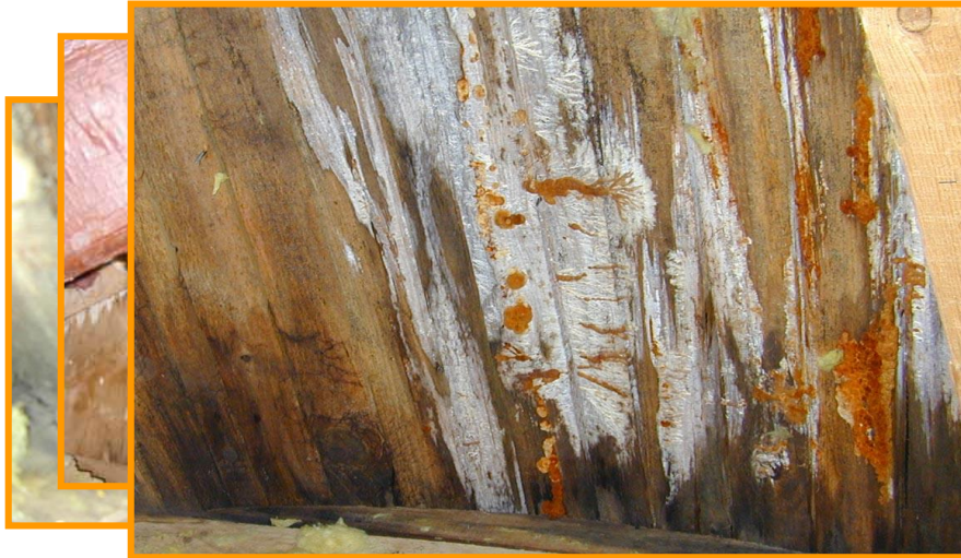
Registered damages caused by wood-decaying fungi (Serpula lacrimans) in Germany: 200 Mio Euro/a
