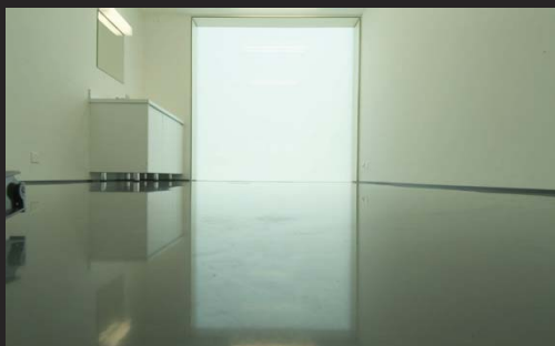
thermal mass for cooling storage and natural light to reduce internal heat gains
