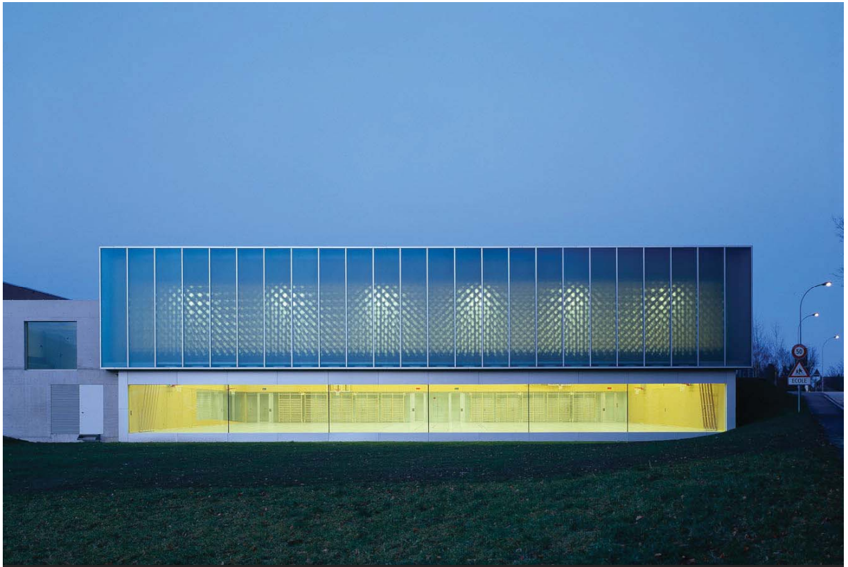
100% glazing in the East en in the South facades , with no visible opening
