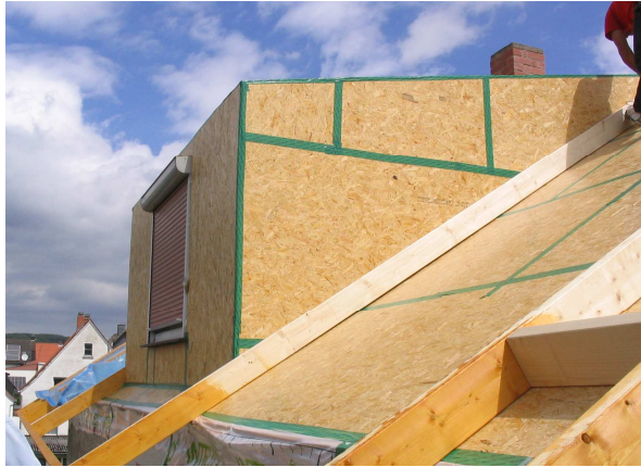
Abb.5: Gaubenanschlüsse
