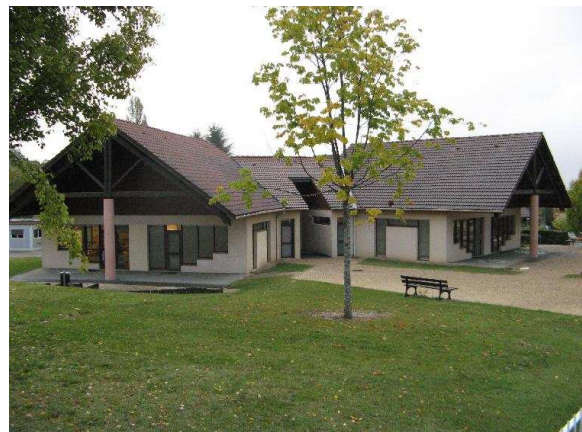
Figure 2 - Primary school building.
