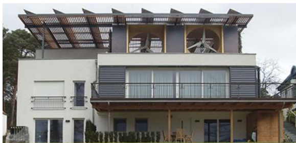
Fig. 9: test and reference building implementing in-house micro-wind-turbines, PV, CO 2 -heat-pump and 12m 3 heat storage and management system
