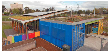
Figure 1b - The Venny photo (source: City of Melbourne)
