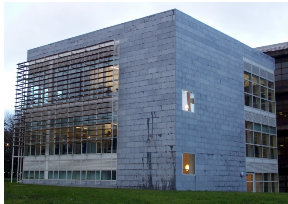
Figure 2 Nursing Library building at the NUI Galway campus
